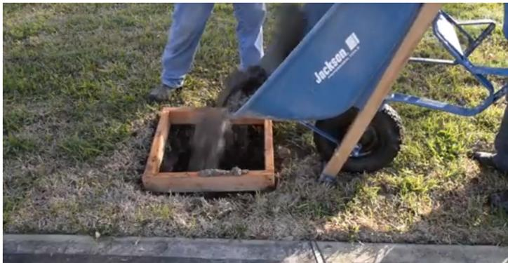
***NOTE: The top of the concrete needs to be level with or higher than your playing area to ensure you system will adjust to 10ft regulation height.***
