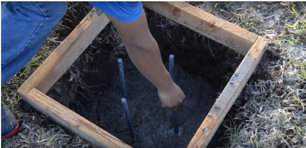
Pour the remaining concrete into the hole until completely full and coming out of the top. Using a trowel, smooth the concrete to your preferred liking.
