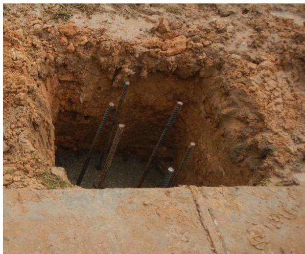
Pour the remaining concrete into the hole until completely full and coming out of the top. Using a trowel, smooth the concrete to your preferred liking.
