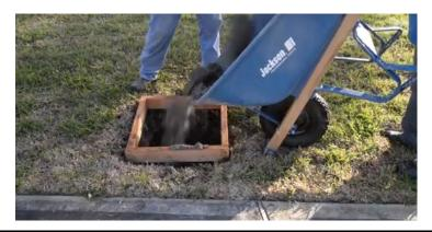
**NOTE:** The top of the concrete needs to be **level with** or higher than your playing area to ensure you system will adjust to 10ft regulation height.
