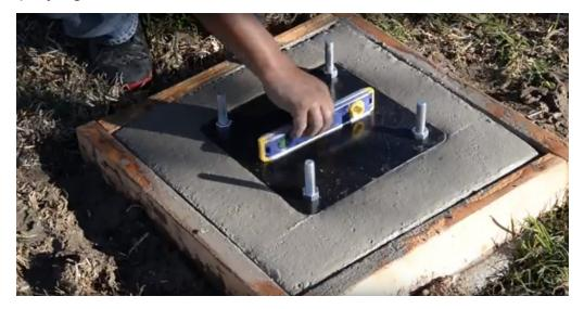
Once completely smooth let the concrete cure. This can take up to a week. Consult the instructions on the concrete bag for curing times and directions.
