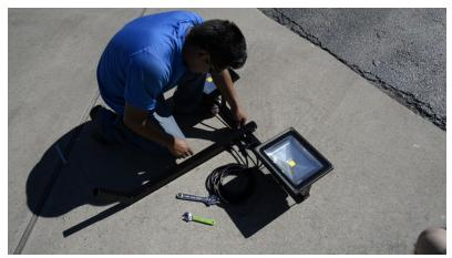
Using the provided Zip Ties (E) secure the electrical wire to the Bracket (C) and Bracket (B).
