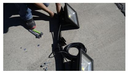
Connect the Bracket (C) to the Bracket (B) using [2] 8mm x 6cm hex bolts (H), [4] 8mm Flat Washers (J), and [2] 8mm Hex Nuts (L). Make sure to tight bolts and nuts.
