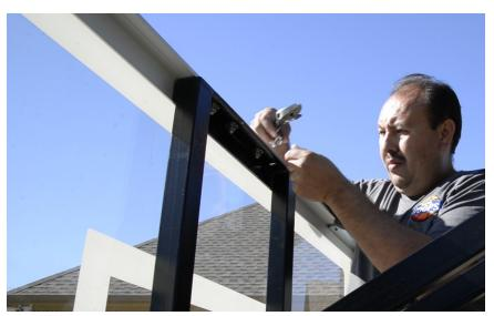
Now install one bolt for your Bracket (A) using [1] 8mm x 4.5cm hex bolts (G), [2] 8mm Flat Washers (J), [1] 8mm Lock Washer (K), and [1] 8mm Hex Nut (L). <u>Do not tighten</u> all the way down just yet.
